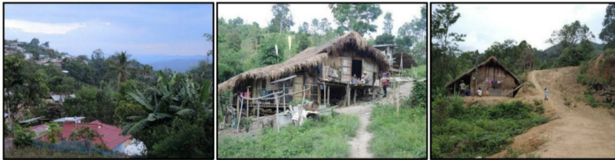
(a) Project setting on the high land
